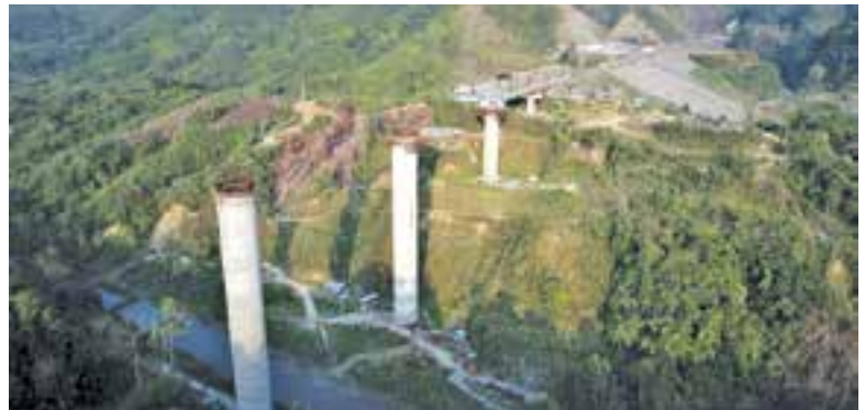
▲ The Ministry of Railways, Government of India, needed to build a 111-km rail line that includes a 141-m-tall bridge in a very active seismic area with high-speed winds and rainfall totals of 3,500 mm per year. (Image courtesy of Indian Railways).
