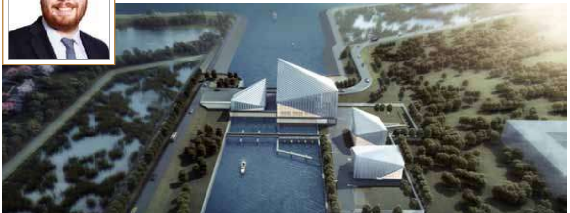
Image caption/courtesy 1: Shanghai Water Engineering was tasked with constructing a pump station with a capacity of 90 cubic meters per second and a sluice gate with a net width of 30 meters. Image courtesy of Shanghai Water Engineering Design and Research Institute Co., Ltd.
