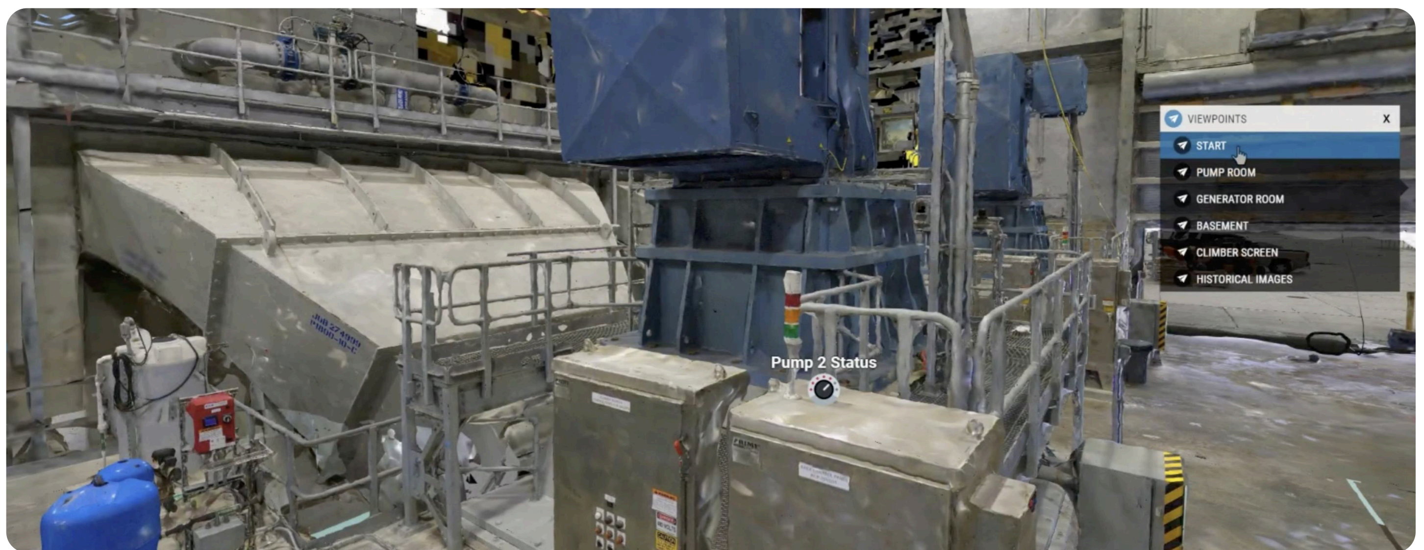
The digital twin enables real-time walkthroughs and condition reviews remotely.
