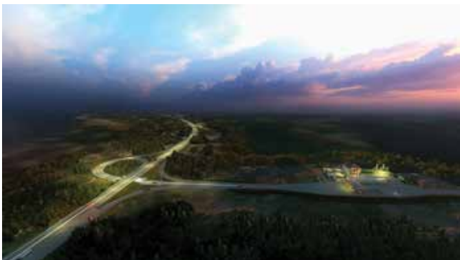
Trans Sumatera Toll Road Project Section Serbelawan-Pematangsiantar (image courtesy of PT Hutama Karya [Persero])
