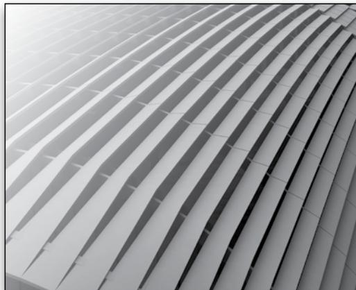
*GenerativeComponents enabled PLP to produce and later verify the fabrication details for the complex roof louvers to minimize the visual effect of the gaps.*
