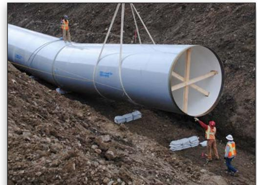
Workers installing the 126-inch diameter buried pipeline.
