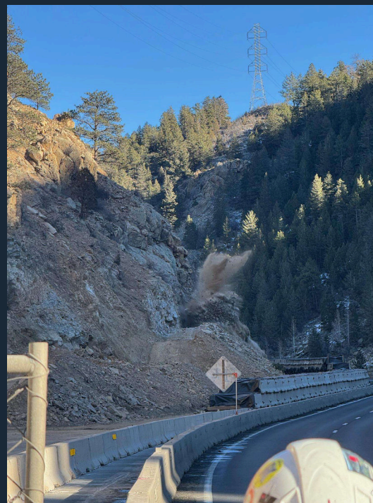
West Section rock blast
