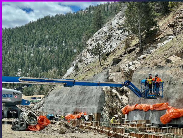
East Section soil nail walls
