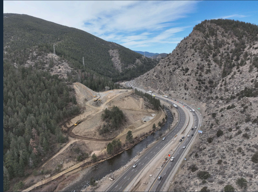
Aerial photo of Central Canyon construction (3/28/25)
