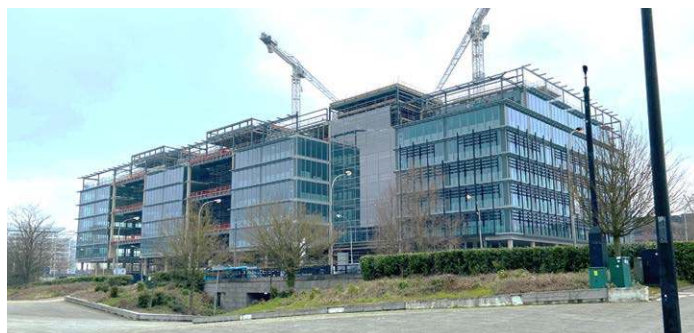
WSP used iterative design to lower the amount of concrete needed by 16,000 tons, save significant material costs, and greatly reduce carbon emissions.
