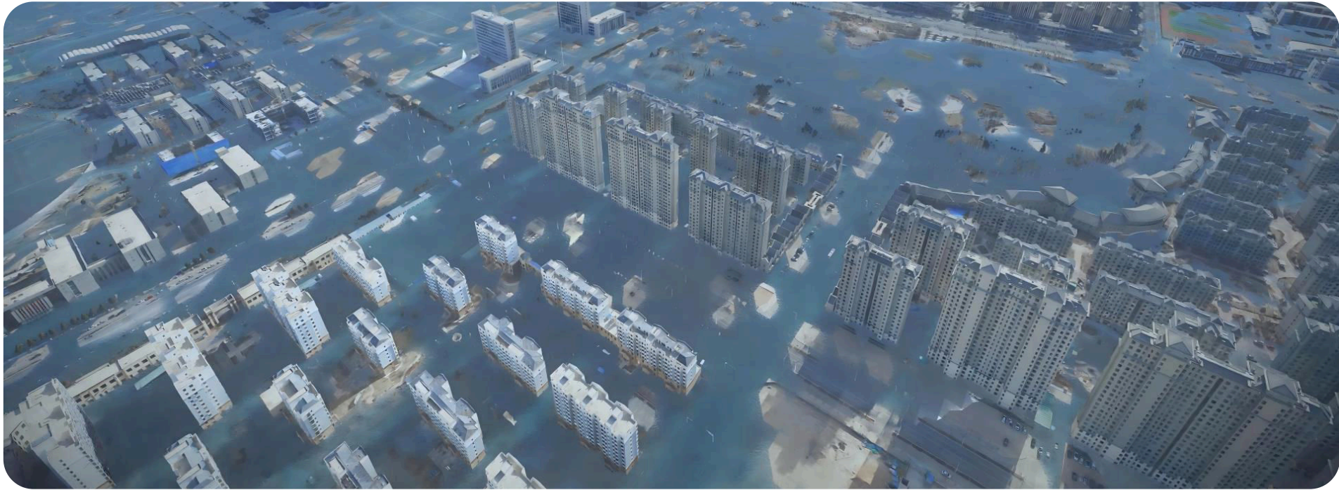
OpenFlows Sewer reduced analysis time for a 30-year storm scenario from weeks to hours, all while accurately identifying overload risks on a key pipeline.
