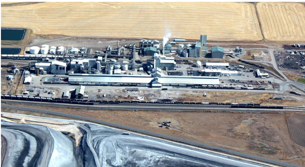
Leveraging the capabilities of AssetWise enabled Itafos to better understand the operating context of their equipment for more sustainable long-term plant operations.
