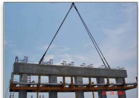
Precast reinforced concrete caps designed with LEAP RC-PIER were used for the majority of the spans.
