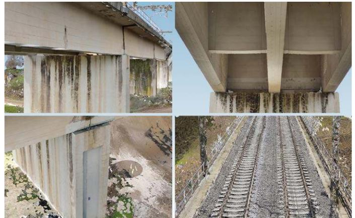
The Borratino viaduct is 1,300 meters long and made of reinforced concrete with 50 spans, making it difficult to efficiently integrate the data from several different technologies in sufficient detail.
