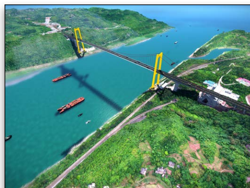
CRCTDG selected ContextCapture to process unmanned aerial survey data and establish a highly precise 3D model.
