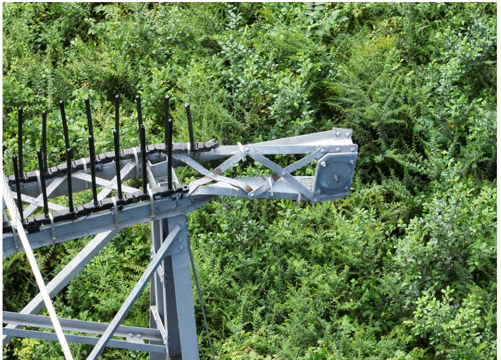
Detailed finite element and wind analysis helped Osmose determine the current state of assets and how they could be rehabilitated.
