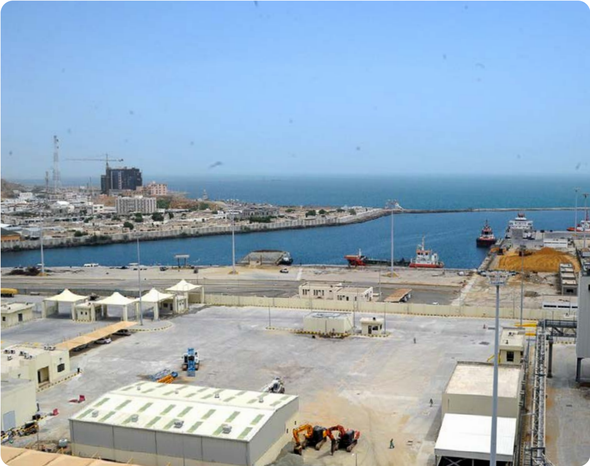
Food security warehouse (bottom left) at Jazan City Port
