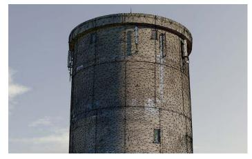
The automatic crack detection technology can quickly detect cracks as small as 0.1 millimeters.
