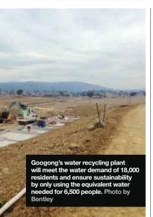
six-meter sloping terrain overlaying rock formations, the AUD 7 million water treatment project required optimum cut-and-fill ratios to minimize costly rock excavation for the underground piping and services.
