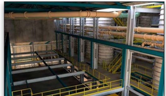
Redundant pipework was color coded in the model and helped reduce the overall load on the building.
