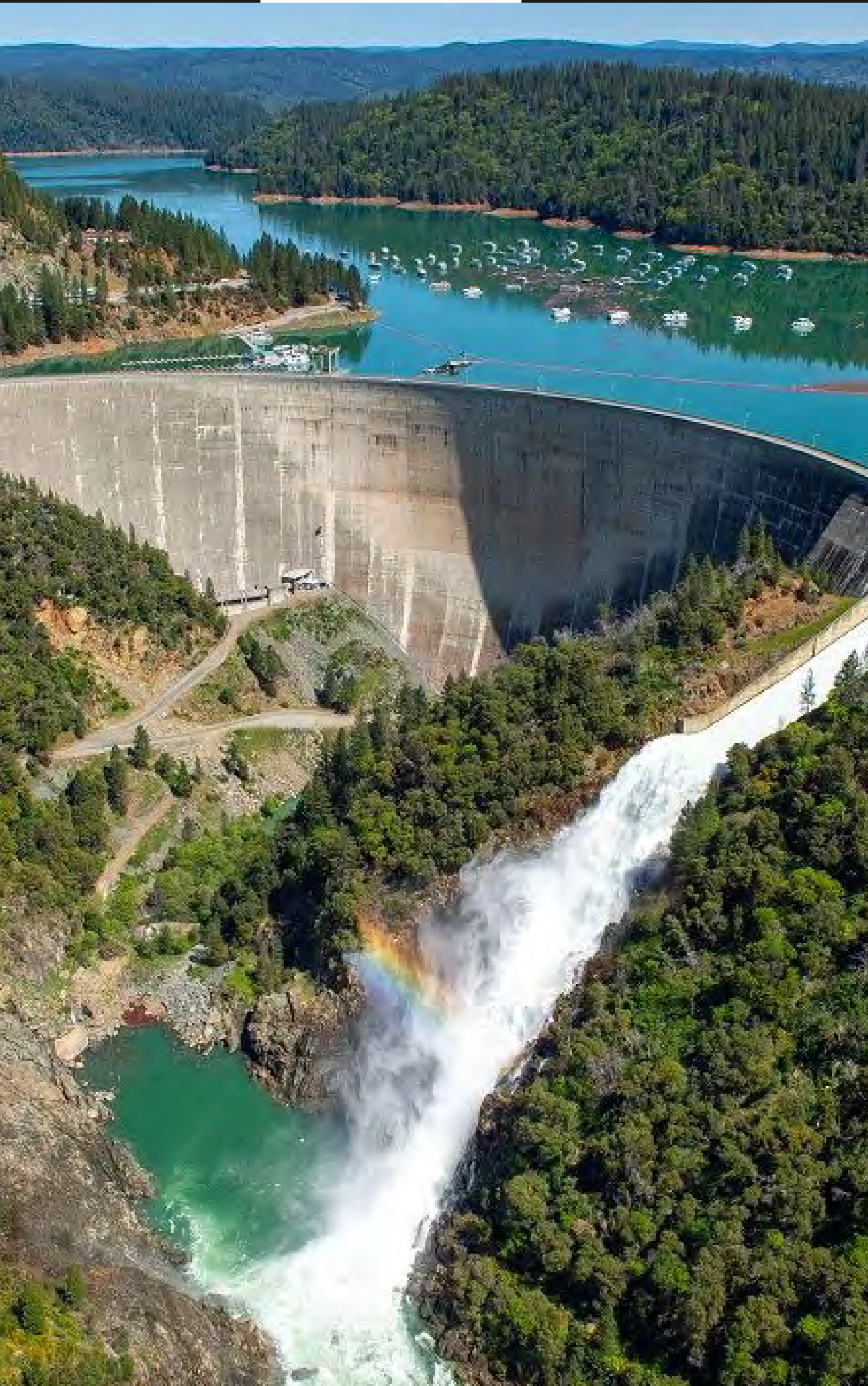
Image courtesy of Yuba Water Agency
